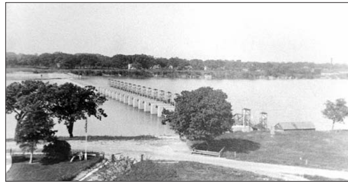
Dam across the Rock river in rock Falls.
