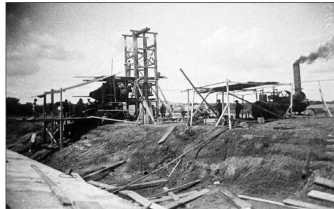
Construction on Culvert 41.
