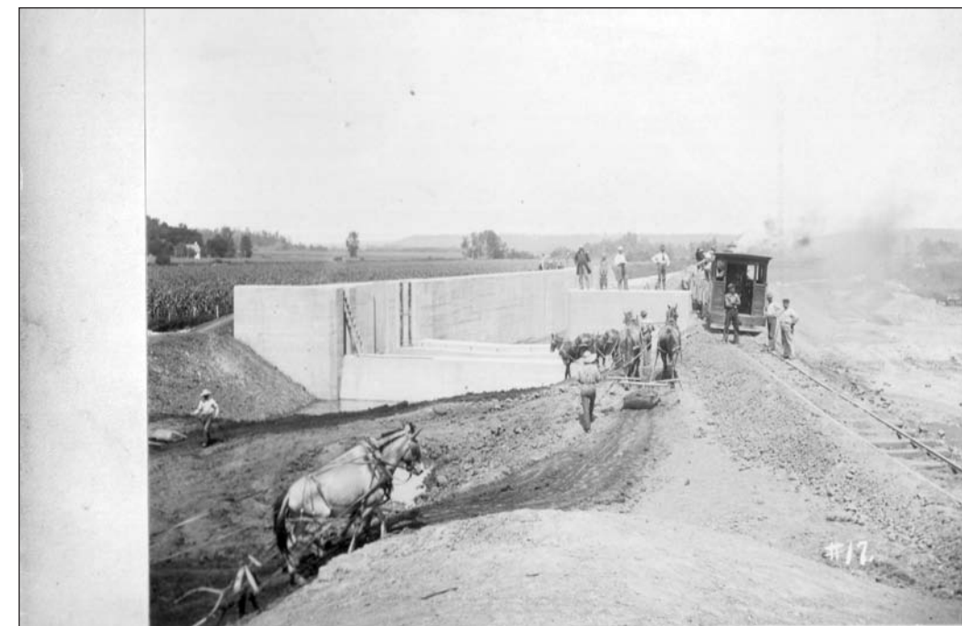
Two "eras" overlap with the horse drawn earth scrapers forming the Canal prism at Lock 5 while the iron horse steam engine brings materials to the workers at the lock.
