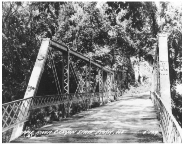
Pratt Pony Truss bridge erected across the South Fork during the late 19th century, looking north. The WPA stencil dates this photo from the later 1930s. The bridge was demolished shortly after that time. (Photograph from State Park files)
