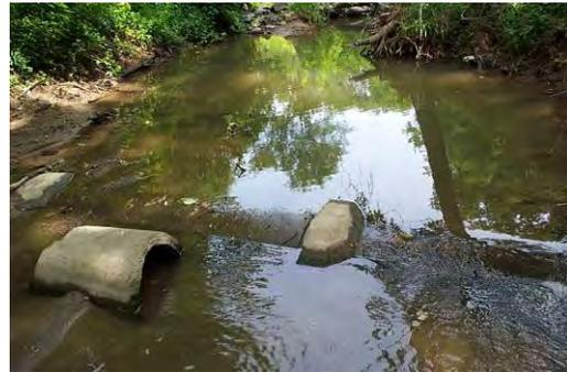
Exposed sanitary pipe in Bull Creek that was originally installed 2-3 feet below the streambed.
