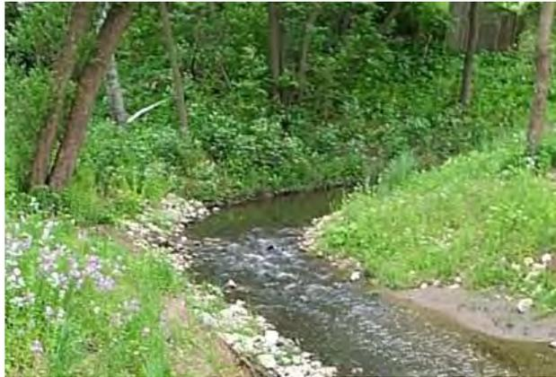
An artificial riffle installed in a restored section of Bull Creek to control incision and improve water quality and habitat
