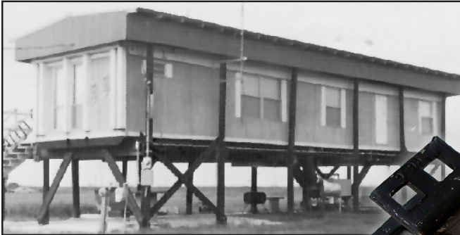
Manufactured Home Showing Cross Bracing and Foundation
