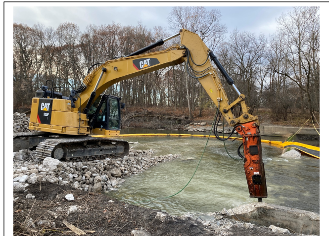
Touhy Avenue Dam Removal
