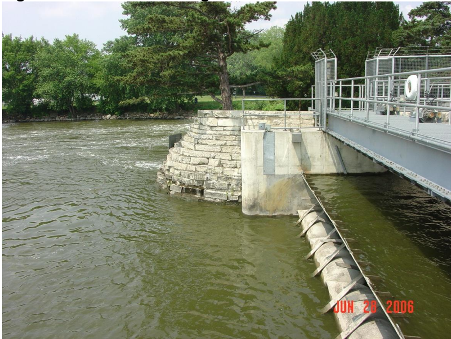
Figure 7: Stratton Dam Hinged Crest Gate
