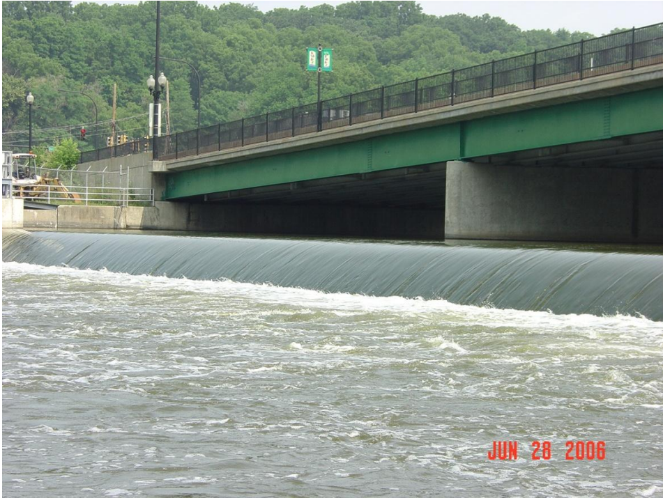
Figure 13: Algonquin Dam Spillway
