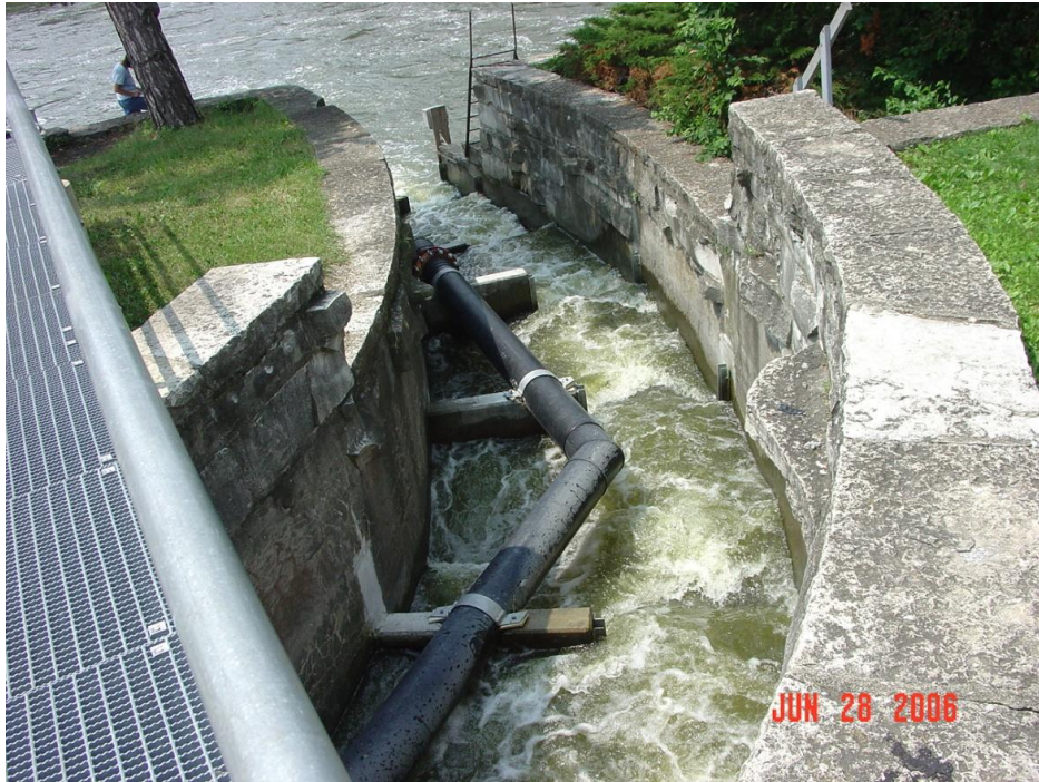
Figure 5: Downstream End of Stratton Dam Fish Ladder
