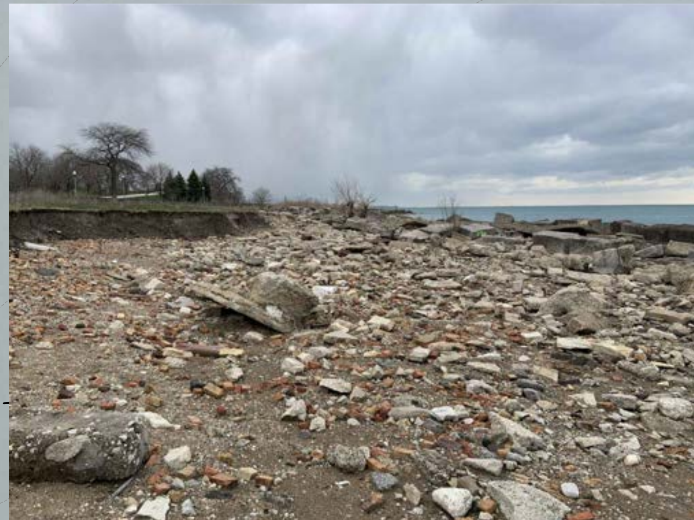
PHOTO B EXISTING DAMAGED PARKLAND, AREA OF ACTIVE EROSION AND DEBRIS
