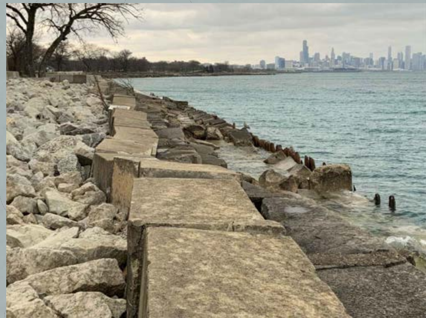
PHOTO A EXISTING DETERIORATED REVETMENT WITH RIPRAP
