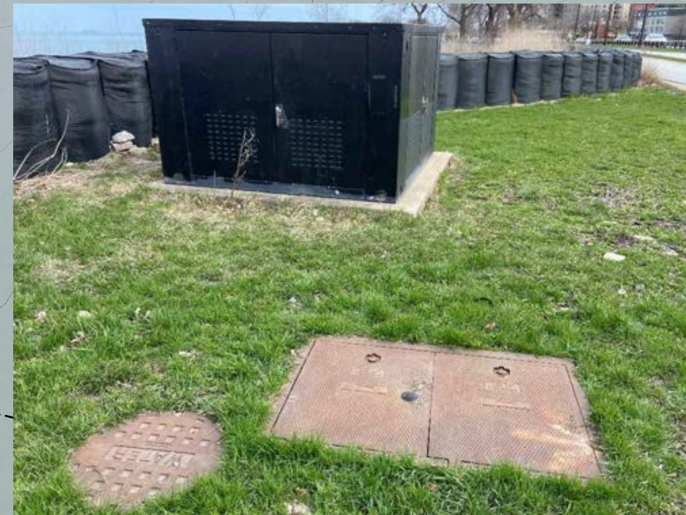
PHOTO C EXISTING (DISUSED) WATER IRRIGATION INFRASTRUCTURE WITH METER VAULT
