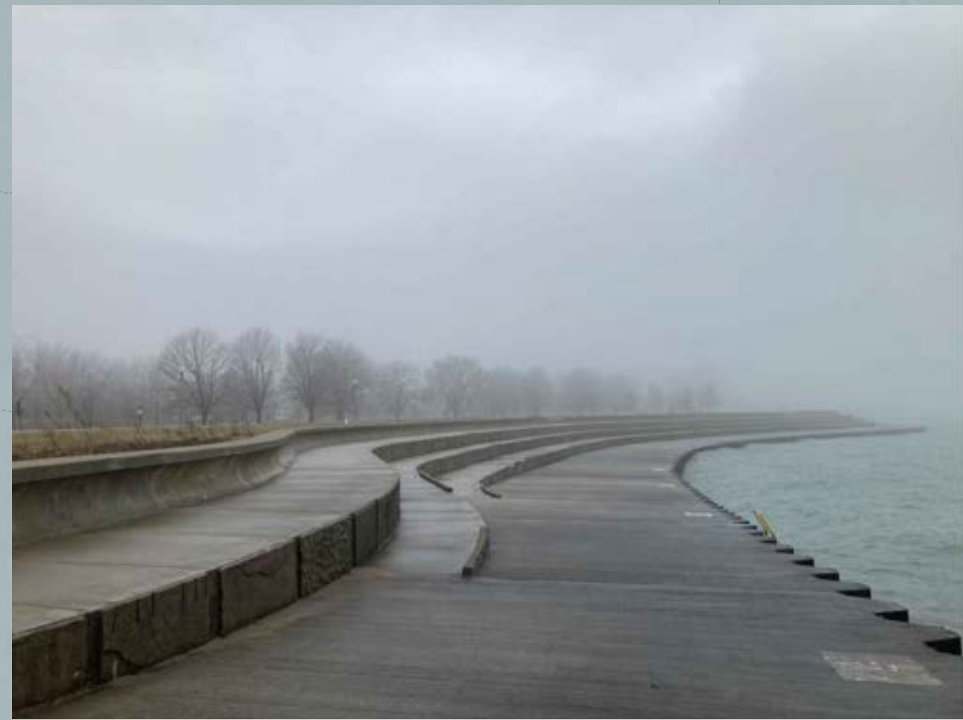
PHOTO A EXISTING STEPPED CONCRETE REVETMENT
