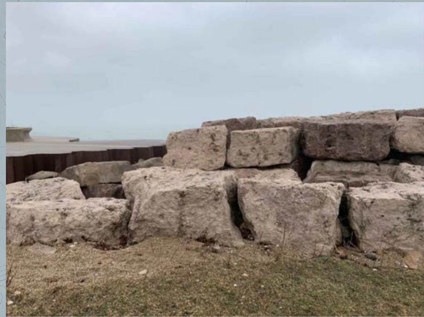
PHOTO B EXISTING ARMOR STONE TERMINATION STRUCTURE
