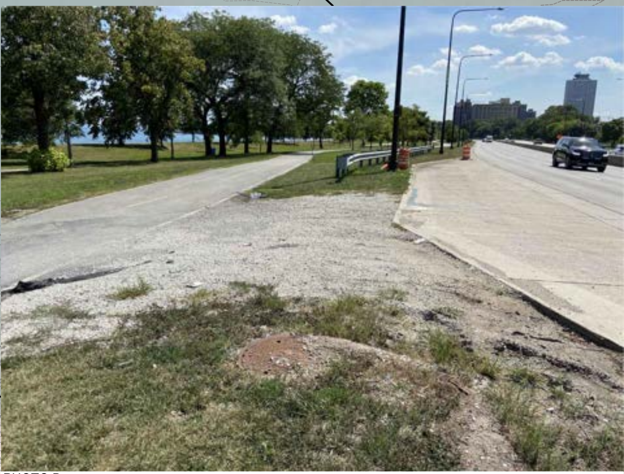
PHOTO B EXISTING DUSABLE LAKE SHORE DRIVE MAINTENANCE ACCESS POINT
